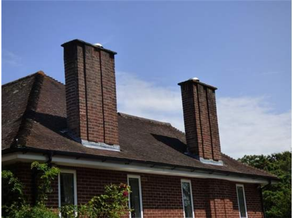
Right side chimney stacks
